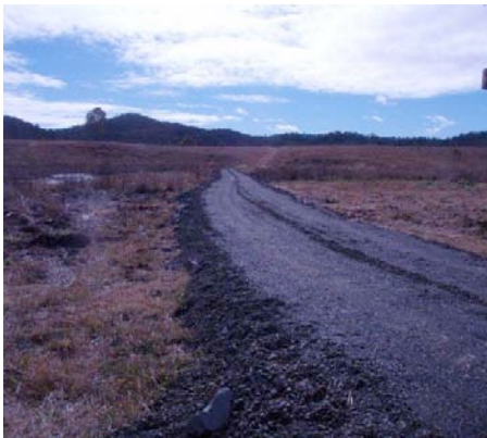
Road upgrade at Stewartdale
